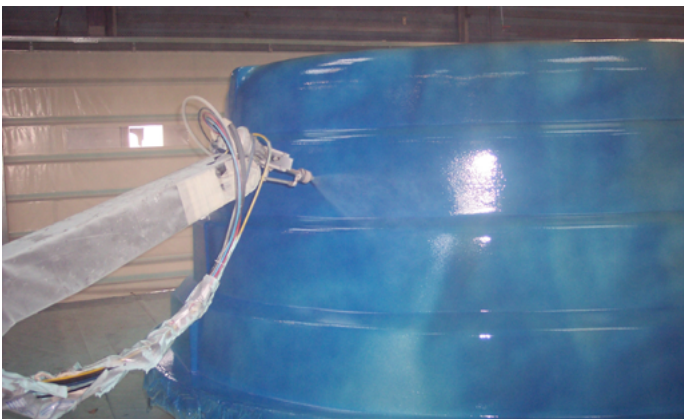
PISCINES IBIZA – Robot spraying of Barrier Coat
